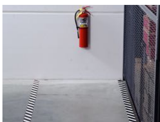
5. Colour-code areas to be kept clear for safety and compliance.
